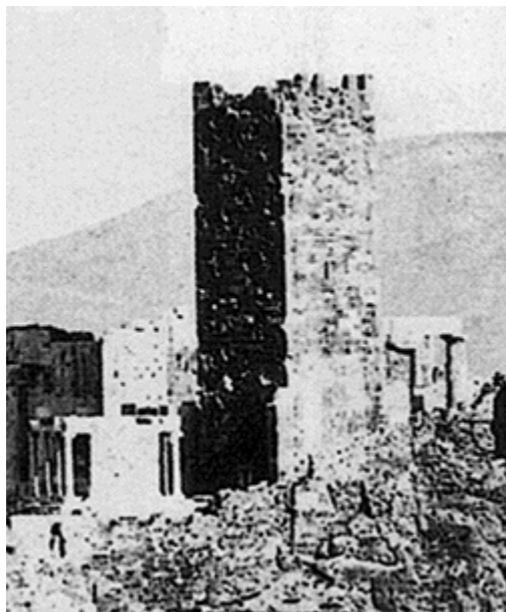
Fig. 7.43. A close-in of a photograph dating from 1865. The mediaeval Ottoman tower
