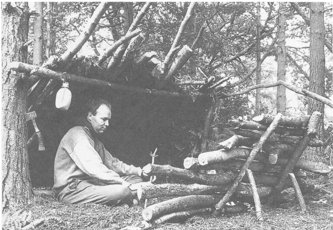
The open-fronted lean-to is quickly and easily constructed and can be used in cold weather although it relies for its warmth on a reflecting fire at the entrance and walls at both ends to exclude draughts.
